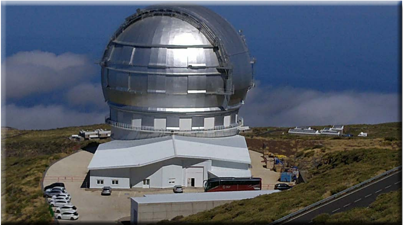
Figure 3: Dome housing GranTeCan. The dome is approximately 100 ft (30 m) in diameter. (photograph by Jürgen Winterberg)
